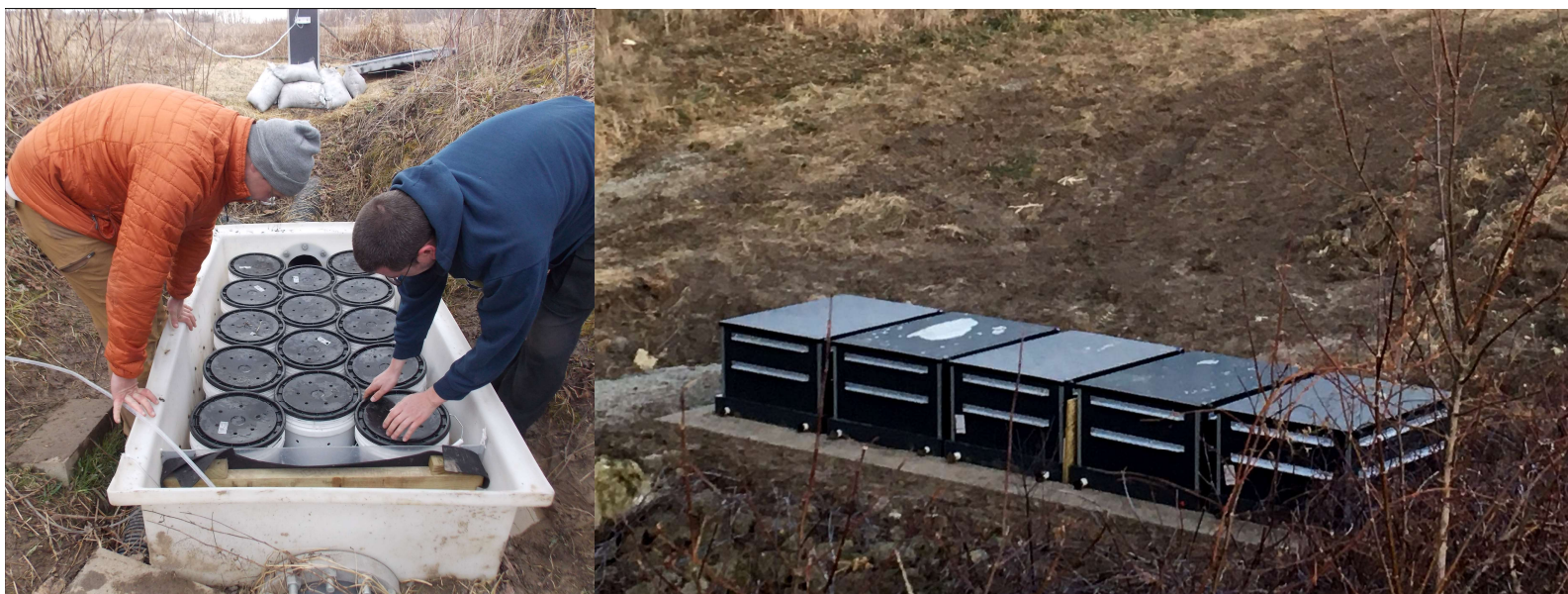
Figure 2. First prototype tile drain CAPTure™ installation (left) and a modular installation of CAPTure™ boxes manufactured by AgriDrain™ (right).
